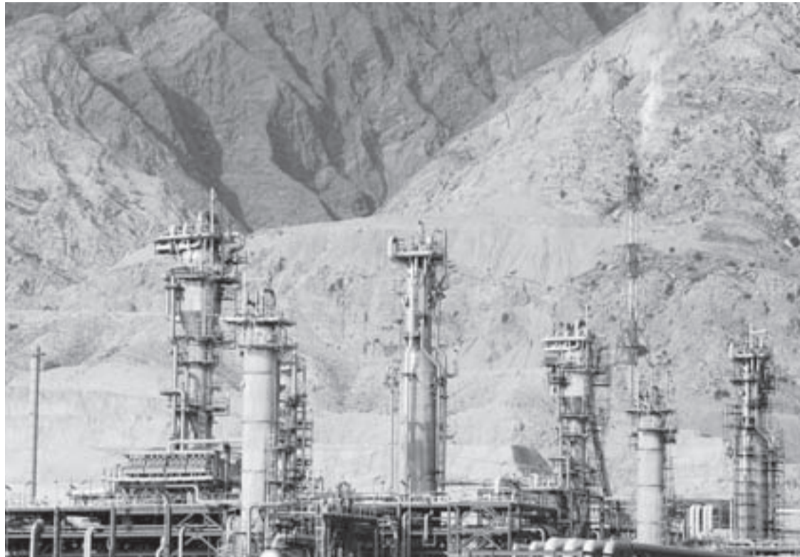
This picture shows a gas refinery at the South Pars gas field on the northern coast of Persian Gulf in Asalouyeh, Iran. With a six-month deal in place easing sanctions as Iran negotiates a final deal with world powers, the government hopes to draw international investment to the natural gas field to spur its production. (AP Photo/Vahid Salemi)
